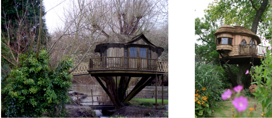
Image 2. Showing Tree Houses Supported Using Timber Bracers.
